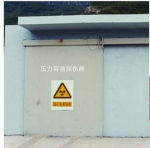
● Testing room outside view
